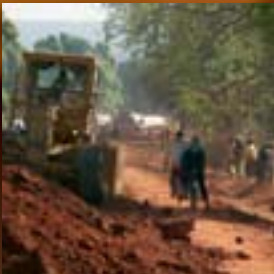
Cat Motorgrader in action in Chad levelling the road.
