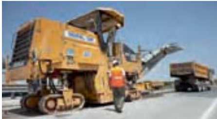
KM 142 A PM200 paver at work
