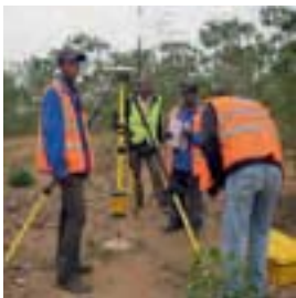
Installation, set up and calibration of the AccuGrade systems and base station was accomplished in just five days.
