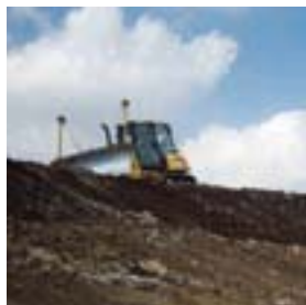
A D6K hard at work restoring a landfill site to its green origins.
