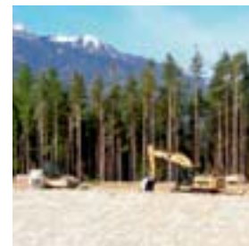
Making the shores of an artificial lake: a 323D near Bressanone.
