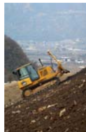
Working at the perfect angle: one of the 6DKs at the Firmiano landfill.
